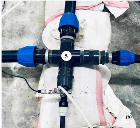
**Fig. 4.5:** (a) Location of the measurement sections around junction 5; and (b) junction 5 (as an example of the service line connection to the WDN).
