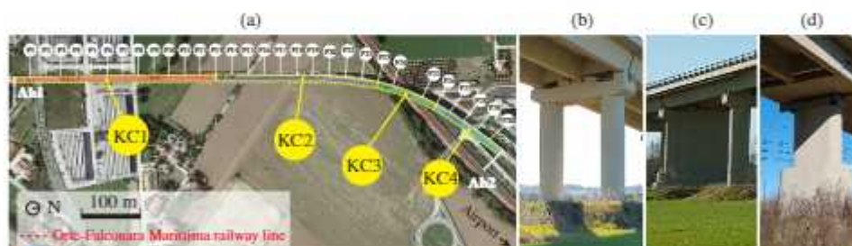
Fig. 1.16: Plan location of the KCs (from Google Maps) (a); view of the column bent piers (b); wall pier (P17) (c); and pier 24 (d).
