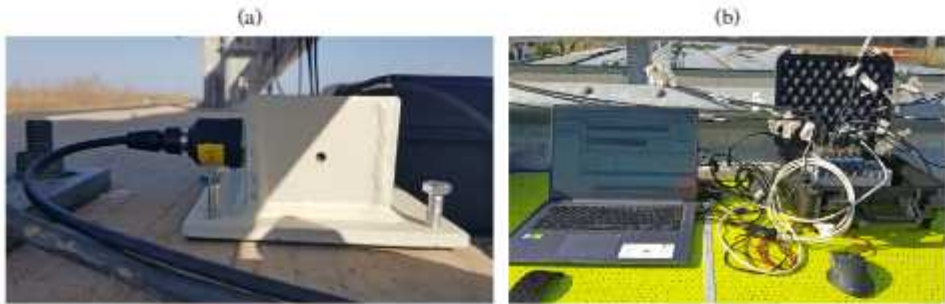
Fig. 1.18: Photographs of an accelerometer fixed to a steel support (a) and the DAQ (b).
